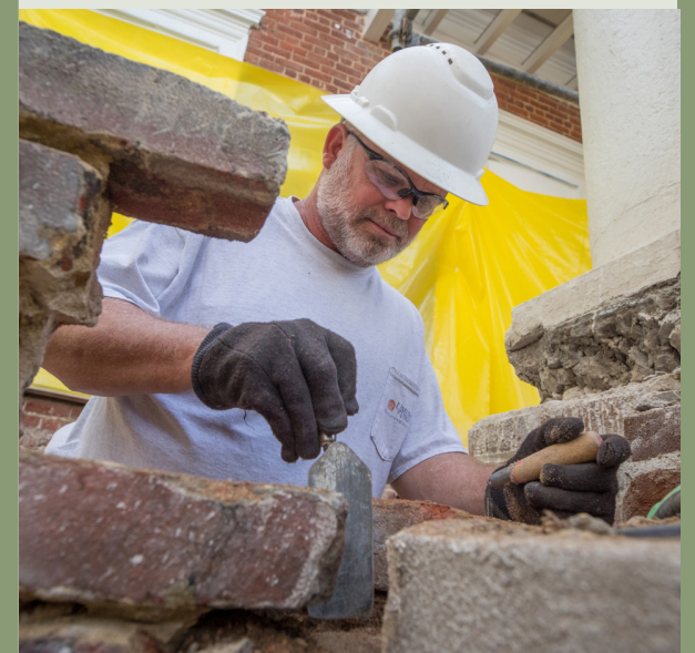
UVA mason reconstructs part of a wall
